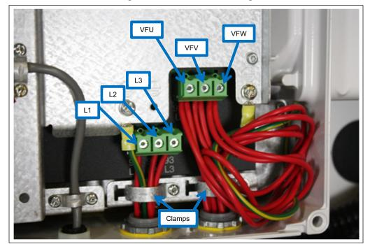
Figure 7.23 VFD Phase Wiring
