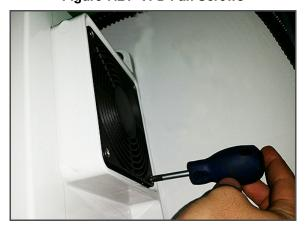
Figure 7.22 VFD Fan Removal
