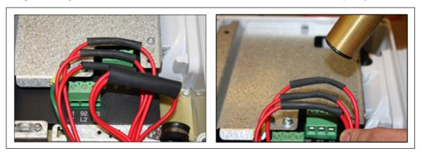
11. While heating the heat shrink tube for a two-to-one butt splice electrical connection, use a needle-nosed plier to crimp the heat shrink tube while heating.
