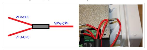
10. Using a hot air gun, shrink the heat shrink tube to insulate all of the electrical butt splice joints.
