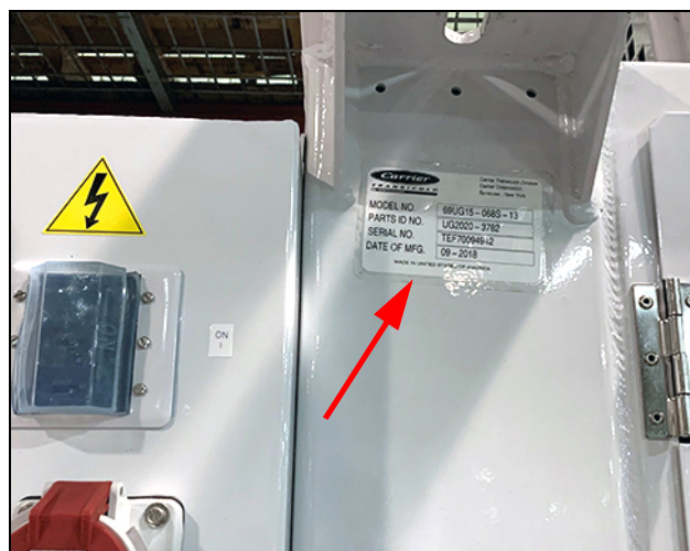
Figure 2.1 Label with Generator Set Identification
