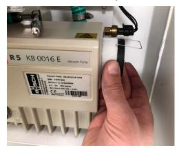
11. Attach the adaptor (818725A) to the filter. Check that the pin of the filter end cap is between 2 fingers and be careful not to get the wire bow between the adaptor and the filter. Gently position the end piece and tighten the 4 screws first with 1 Nm and then with 3 Nm.
