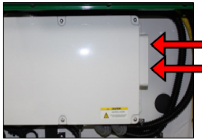
Figure 25 VFD Fan Rotation
