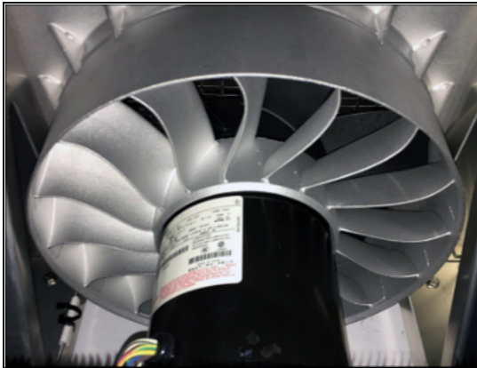
Figure 2 Evaporator Motor and Fan Blade
