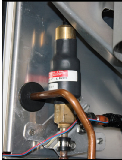
Figure 6 Electronic Expansion Valve (EEV)
